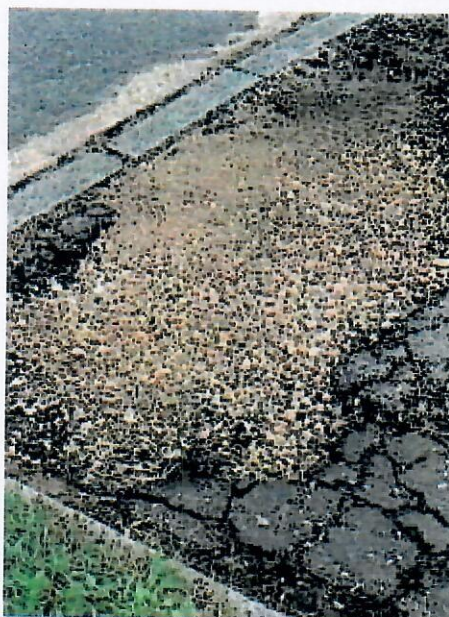
Bowes Drive no 16 Dropped kerb/driveway collapsed
